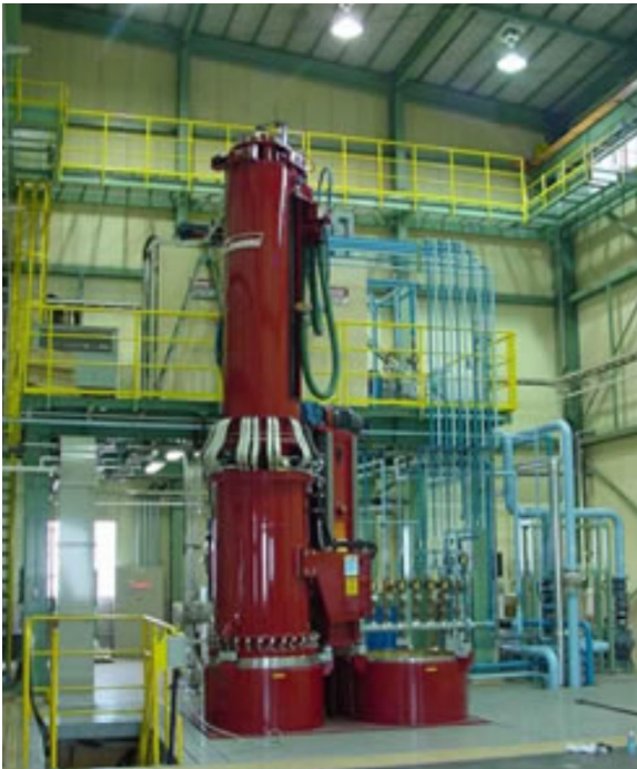
Figure 9: Photograph of the top of a (newly installed) VAR furnace.
